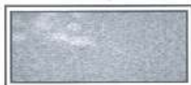
11 / Weathering/Ravelling
